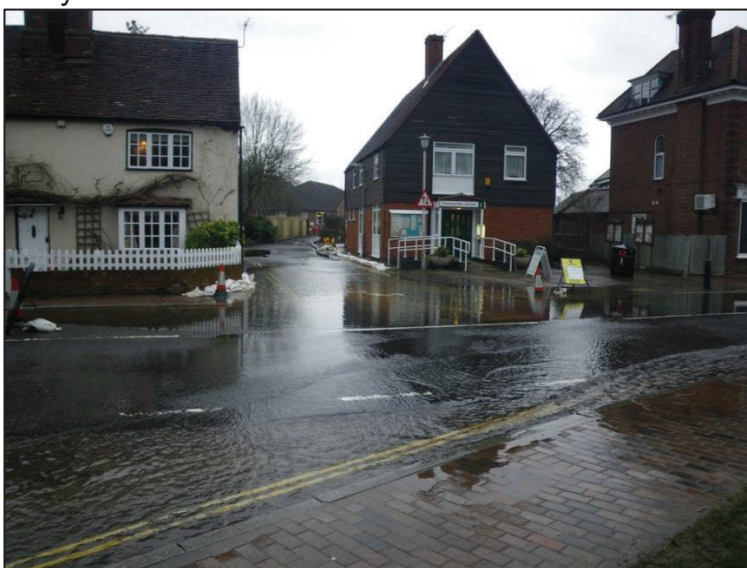
Flooding in Chalfont St Giles, 2014 (Photo supplied by the Environment Agency)
