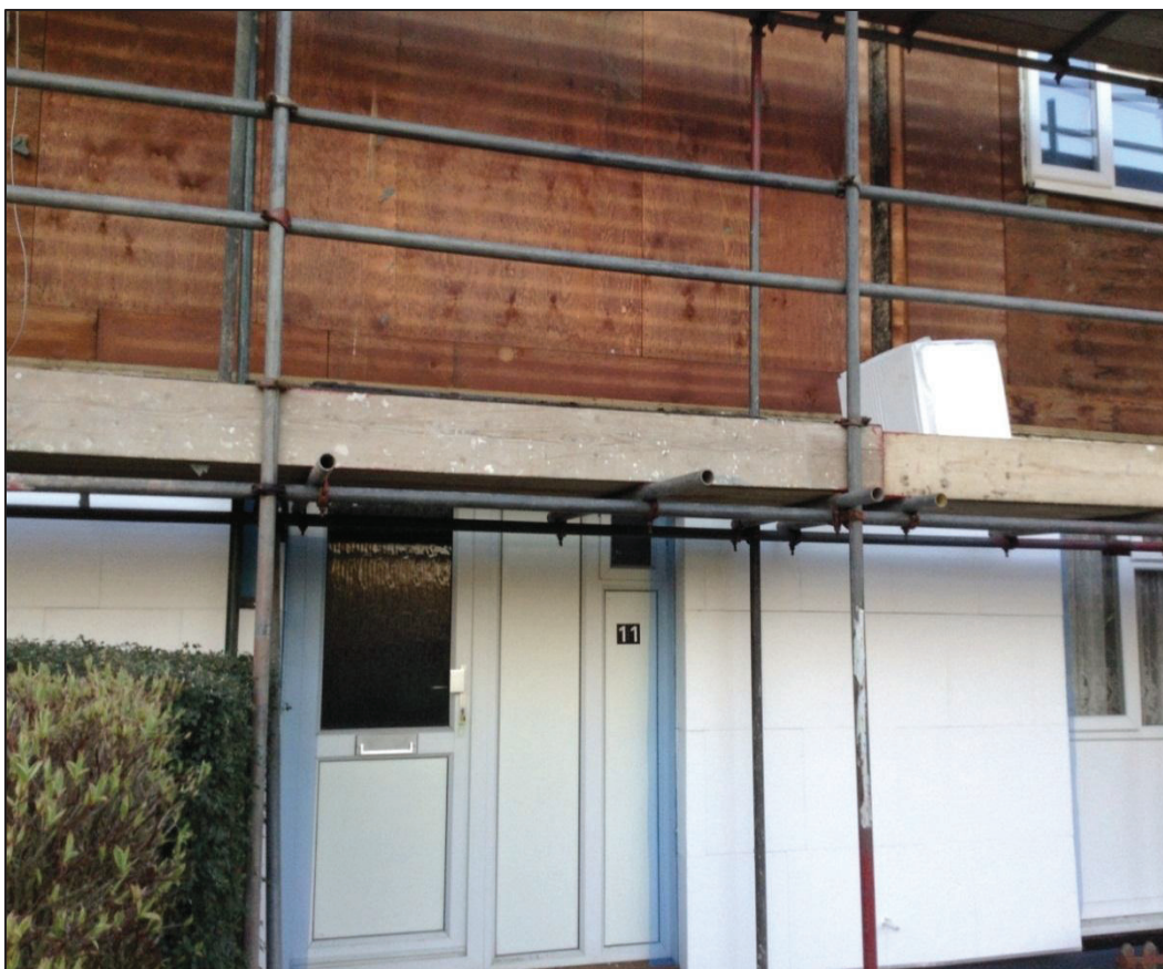
Retrofitting an existing house with external insulation
